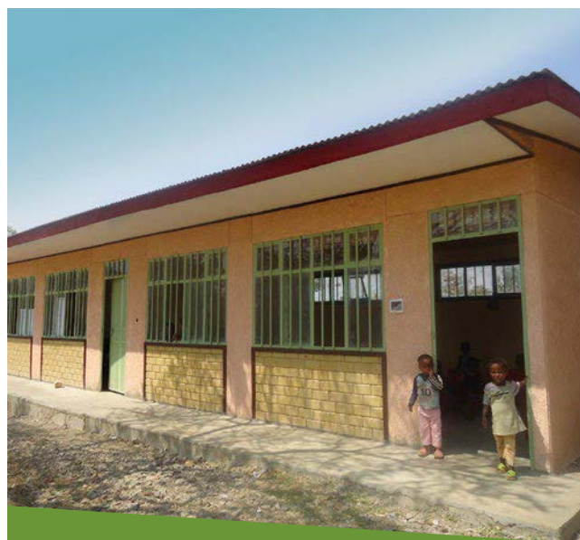
Communities are initiating school infrastructure projects, like this new classroom block in Wonchi District, Ethiopia.
